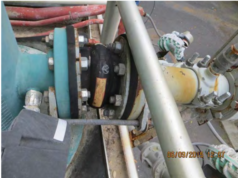
Photo 2-67: Orchard Run WTP Pump Station Deflection of Coupling and Corrosion on Piping
