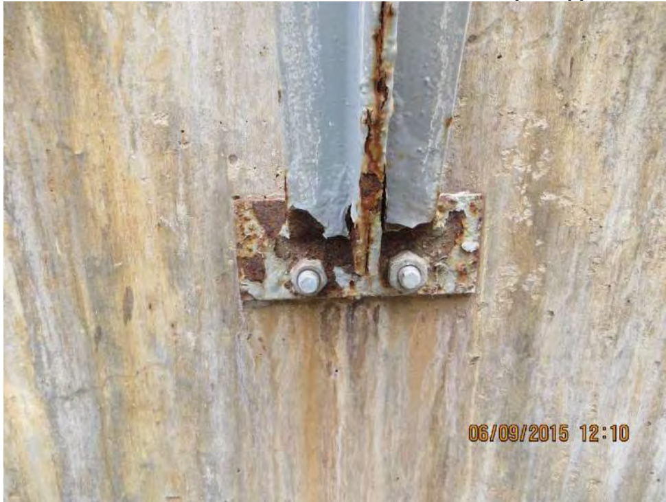
Photo 2-68: Orchard Run WTP Pump Station Corroded Pipe Support Strut
