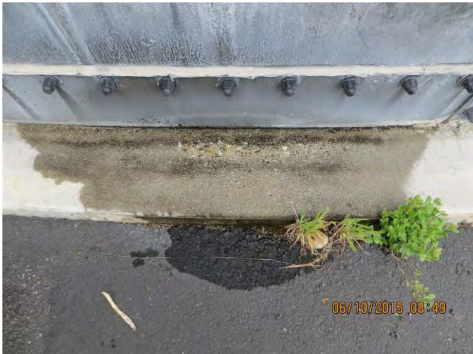
Photo 2-112: Recycled Water Tank – Minor Erosion of Concrete Ring Wall Footing
