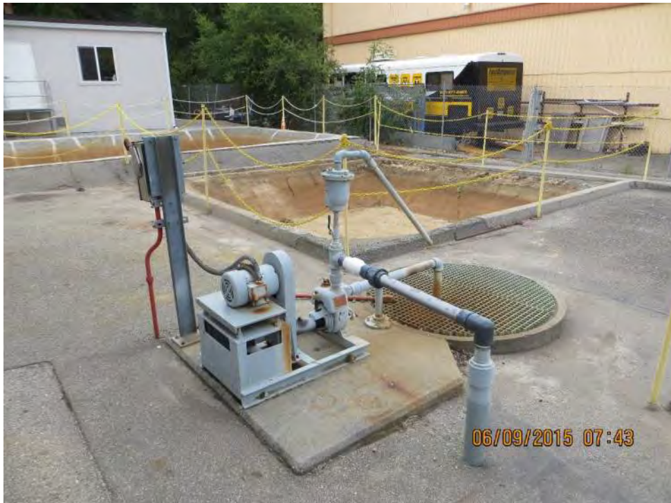
Photo 2-24: El Pueblo Water Treatment Plant Reclaim Pump and Sedimentation Basins
