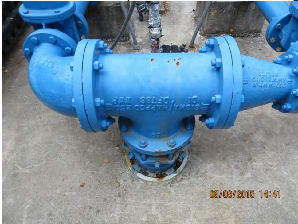
Photo 2-42: Crescent Pump Station Corrosion on Ductile Iron Fitting
