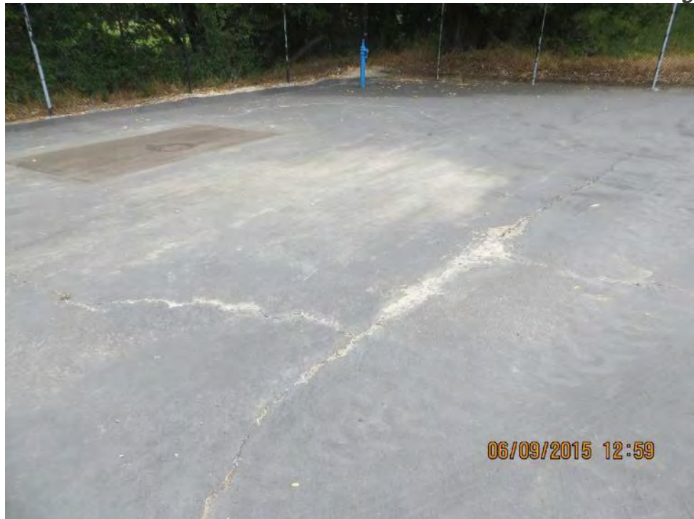
Photo 2-2: Well 3B Site Cracked Paving
