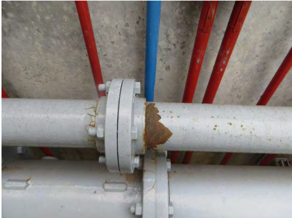
Photo 2-38: Orchard Run Water Treatment Plant Typical Yard Piping with Damaged Coating/Corrosion
