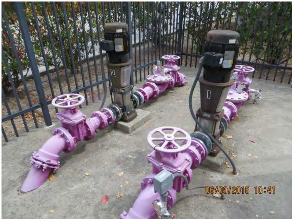
Photo 2-103: Siltanen Pump Station Mechanical Layout
