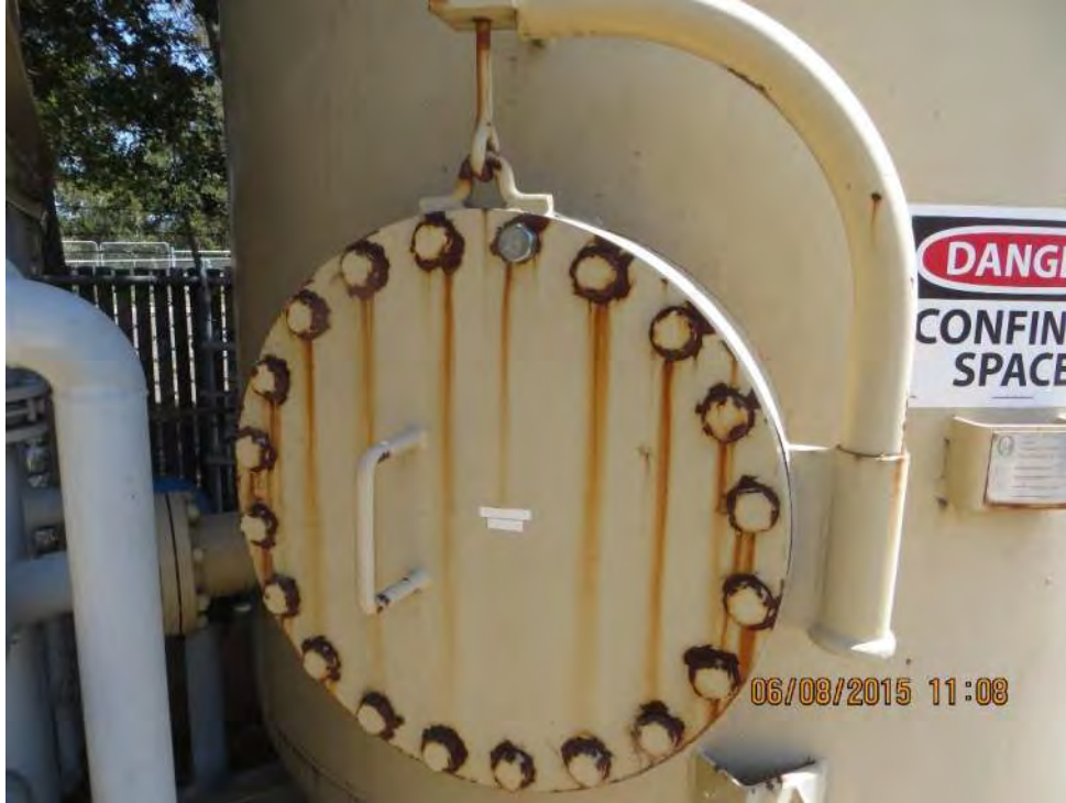
Photo 2-18: Well 9 Water Treatment Plant Corrosion on Manway
