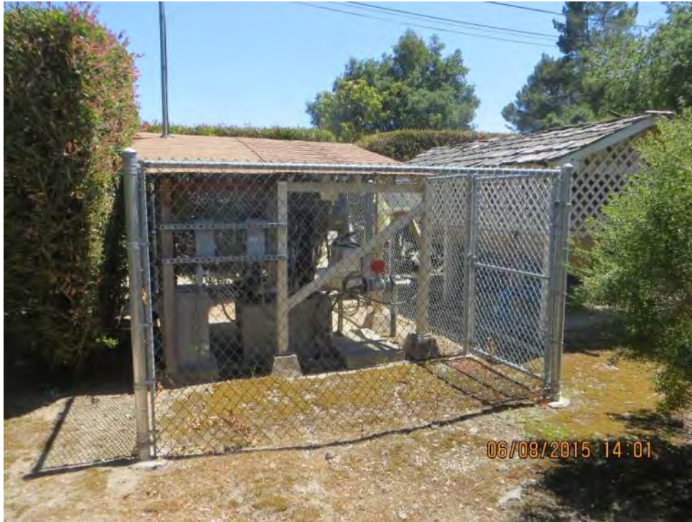
Photo 2-55: Hacienda Pump Station – Unpainted Timber in Background & Corrosion on Piping
