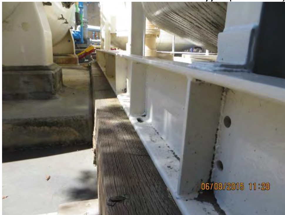
Photo 2-22: Well 10A Water Treatment Plant GAC Filter Timber Support (Un-anchored)
