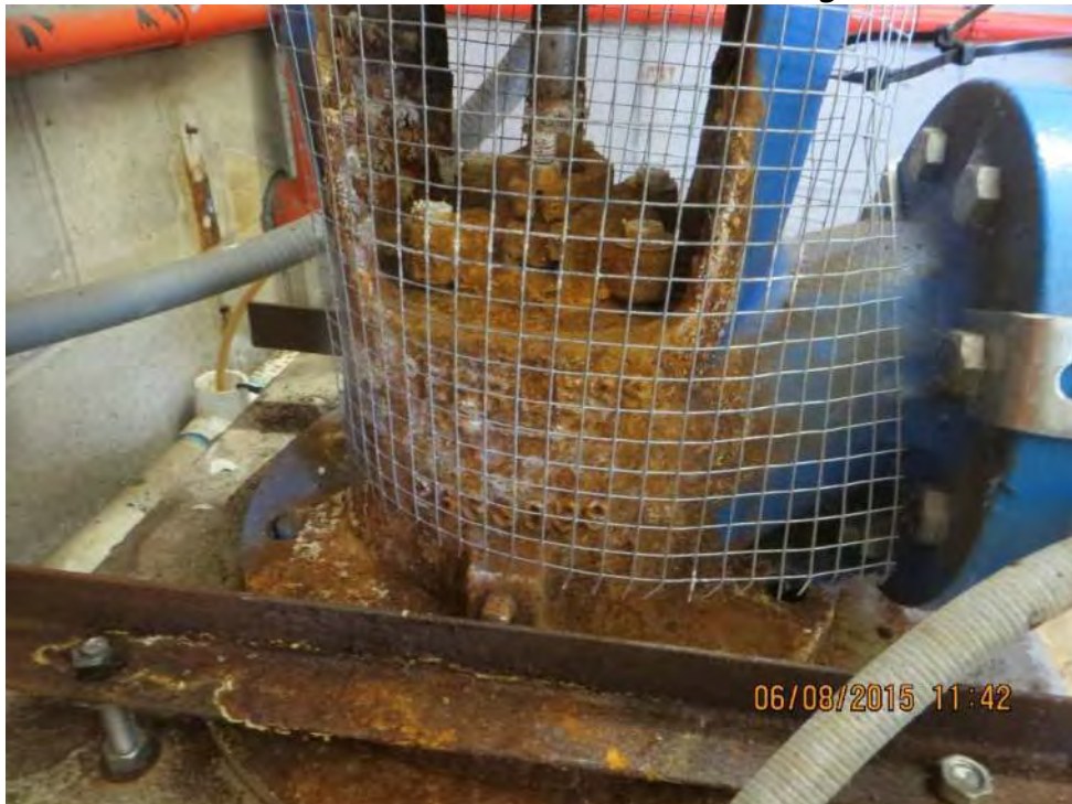
Photo 2-61: Well 10A WTP Pump Station Mechanical Seal Leakage and Corrosion
