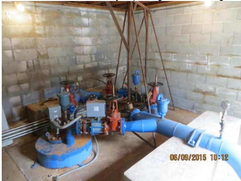
Photo 2-43: Bethany Pump Station Mechanical Layout (Staining on Walls in Background)
