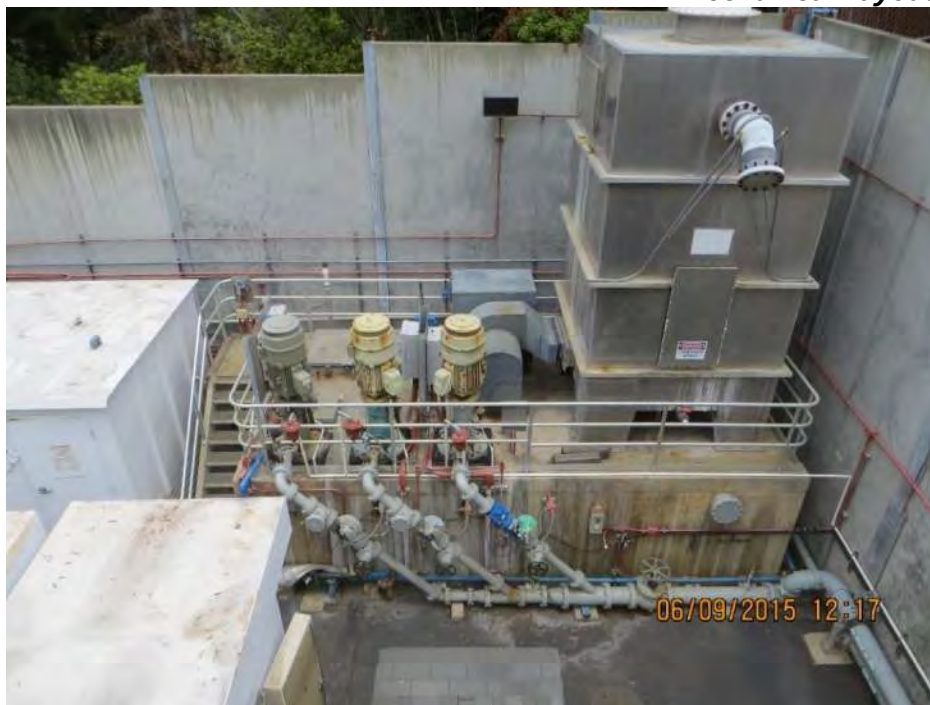
Photo 2-65: Orchard Run WTP Pump Station Discharge Pipe Arrangement
