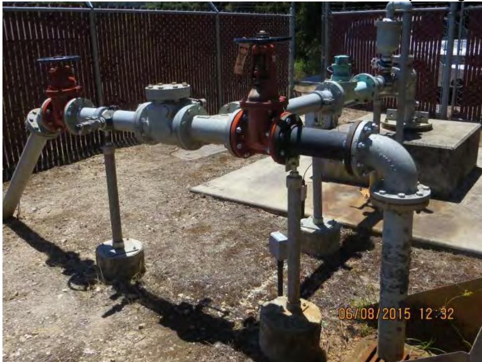
Photo 2-12: Well 11A Mechanical Layout – Exposed Ductile Iron Pipe/Flanges
