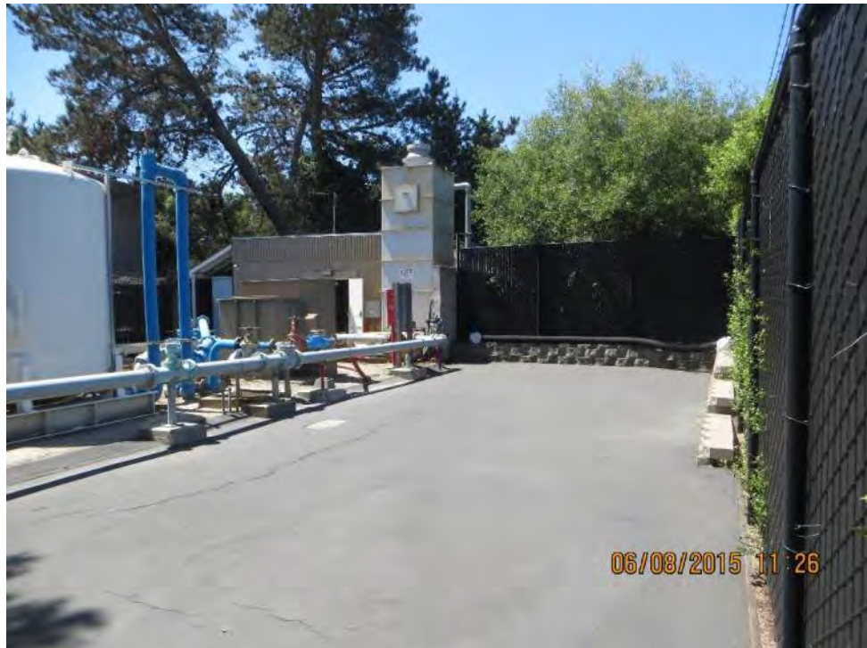
Photo 2-20: Well 10A Water Treatment Plant Chemical Feed Building, Air Stripper and Cracked AC
