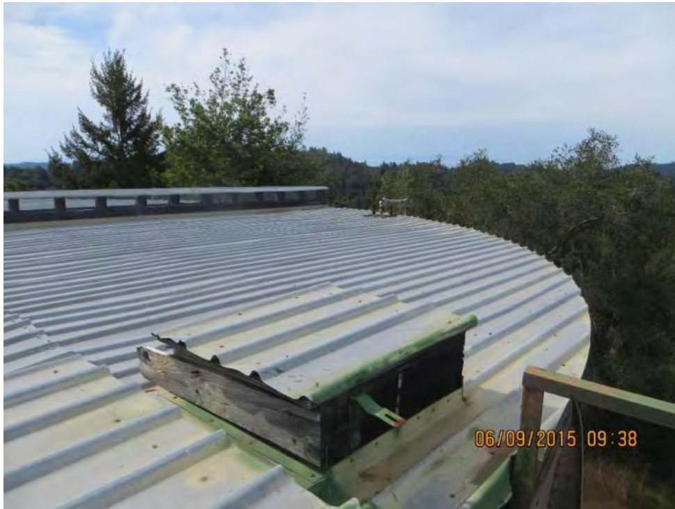
Photo 2-72: Bethany Tank – Corrosion at Gutter/Top Shell Course
