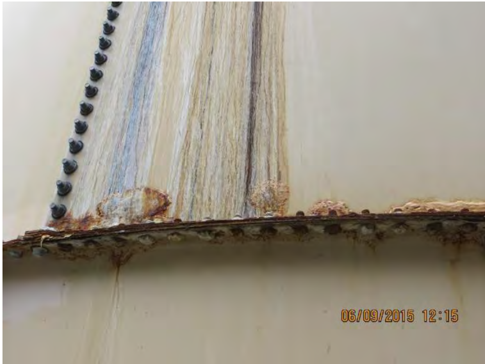
Photo 2-36: Orchard Run Water Treatment Plant Backwash Tank (Corrosion and Past Leakage)
