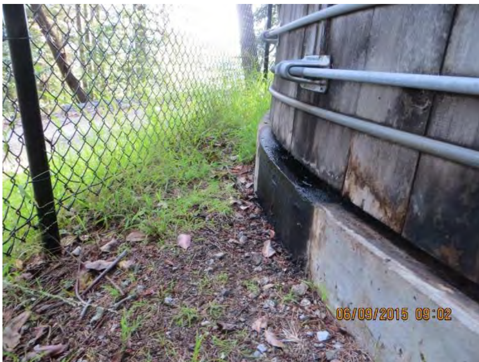
Photo 2-89: Mt. Roberta Tank – Leakage at Tank Base
