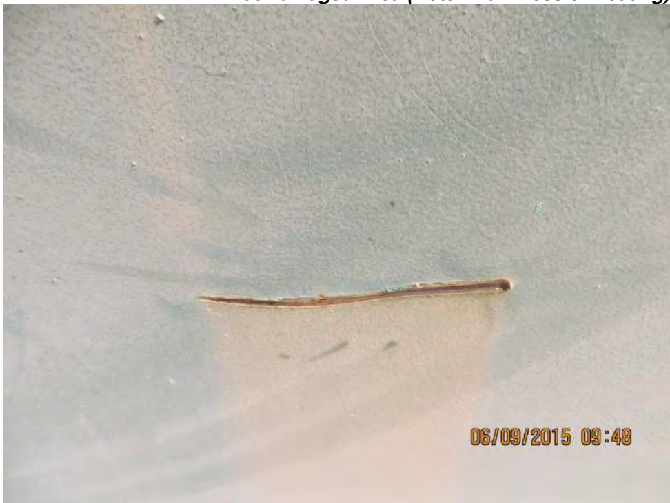
Photo 2-74: Bethany Tank – Spot Corrosion on Tank at Damaged Area (Note Chalkiness of Coating)
