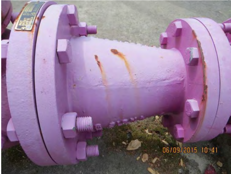
Photo 2-104: Siltanen Pump Station – Corrosion on Pipe Fitting
