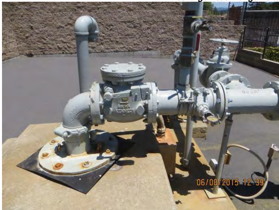
Photo 2-14: Well 11B Minor Corrosion Observed on Discharge Head Flange/Bolts
