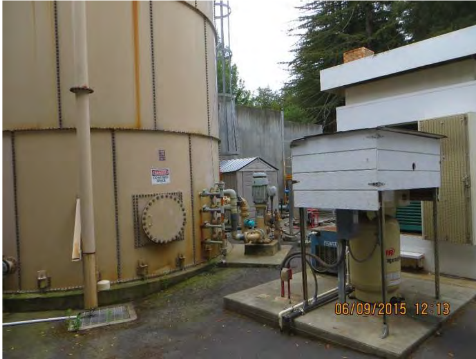
Photo 2-36: Orchard Run Water Treatment Plant Backwash Tank (Corrosion and Past Leakage)
