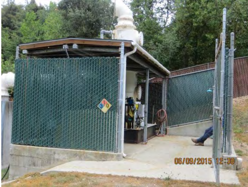
Photo 2-31: Orchard Run Water Treatment Plant Flume Scrubber
