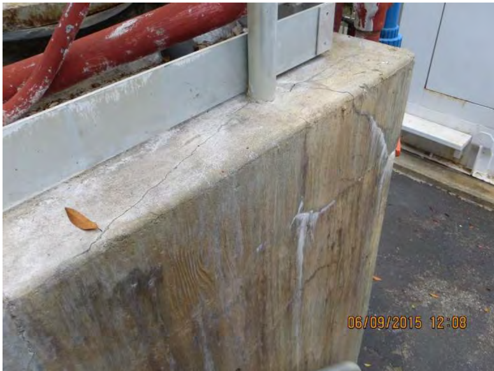
Photo 2-69: Orchard Run WTP Pump Station Cracks in Concrete Clear Well
