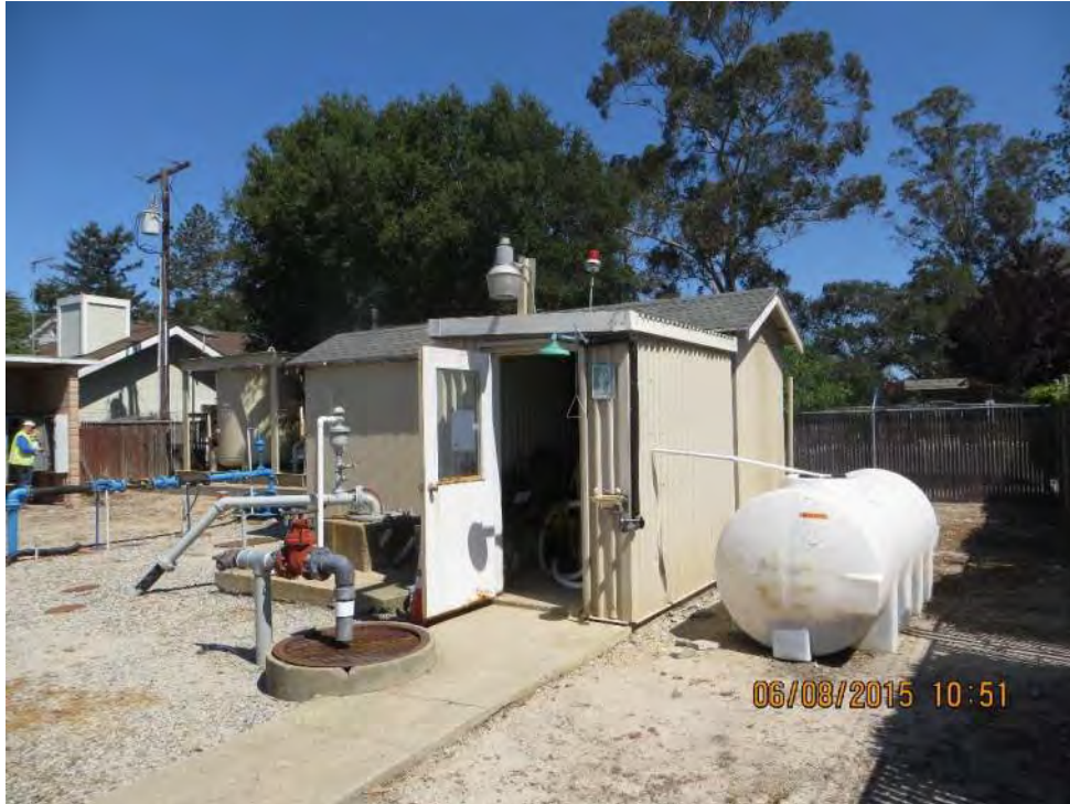
Photo 2-16: Well 9 Water Treatment Plant Chemical Feed Building and Clear Well
