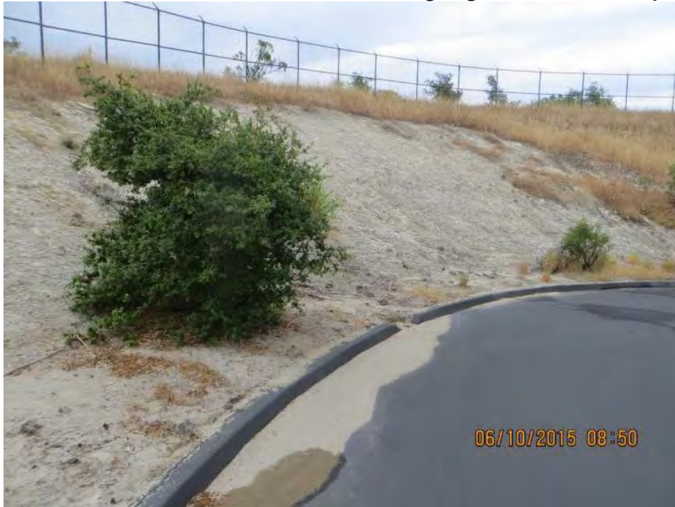
Photo 2-107: Recycled Water Tank – Minor Sloughing/Erosion of Cut Slope
