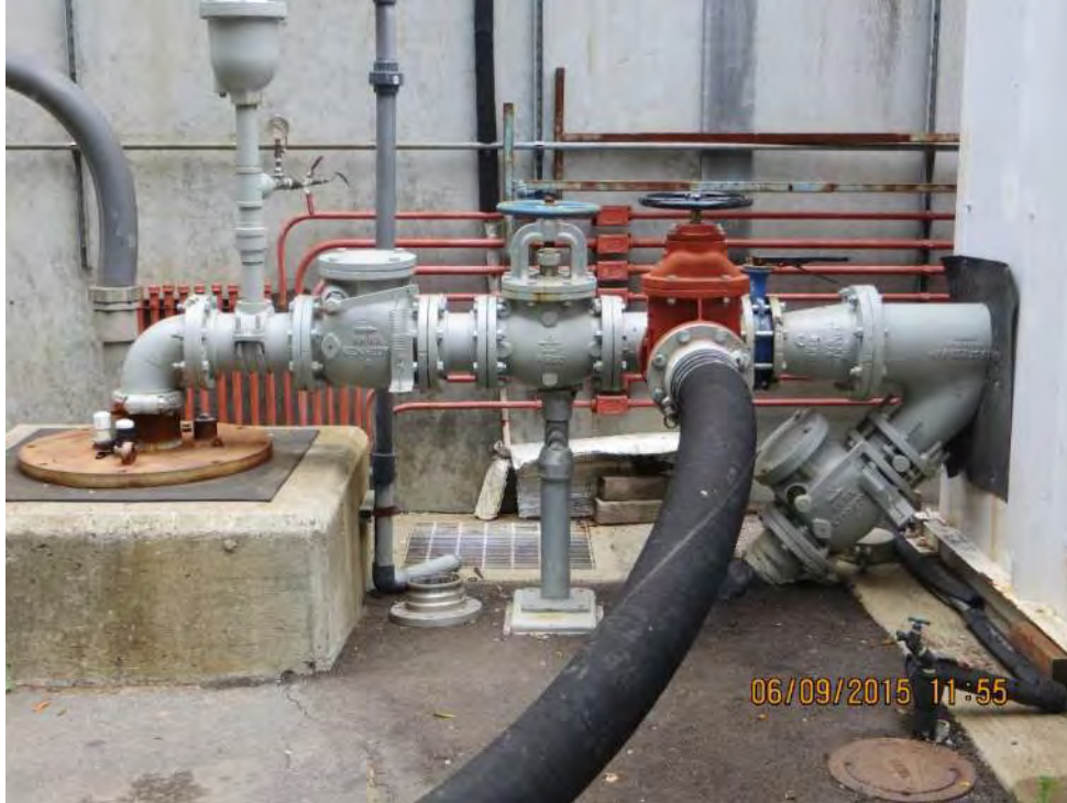
Photo 2-3: Well 7A Mechanical Layout
