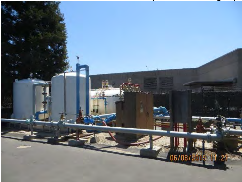
Photo 2-10: Well 10A Exposed PVC Discharge Pipe
