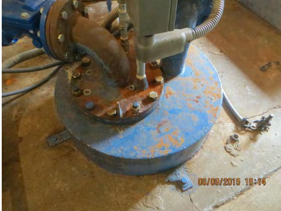
Photo 2-44: Bethany Pump Station Sealed Pump Can Arrangement
