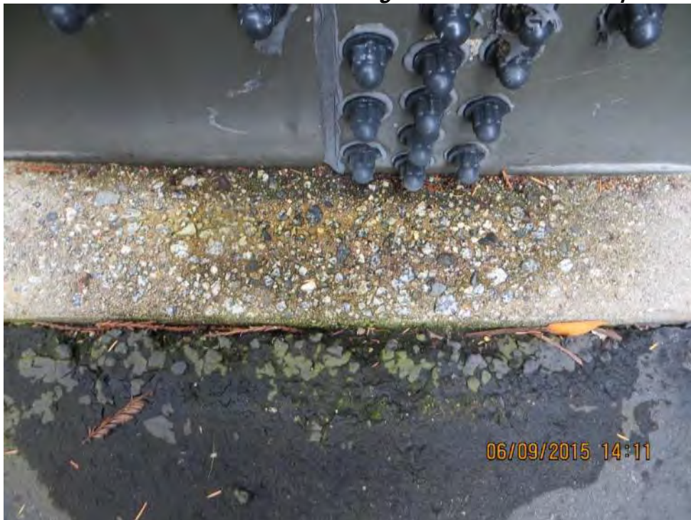
Photo 2-99: Southwood Tank - Erosion of Concrete Ring Wall Surface from Precipitation
