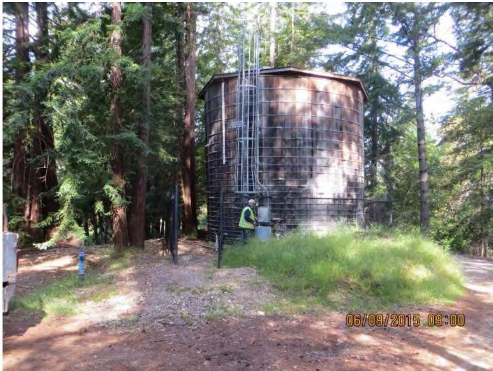
Photo 2-89: Mt. Roberta Tank – Leakage at Tank Base
