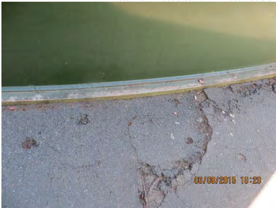
Photo 2-87: Macdorsa Tank – Root Intrusion
