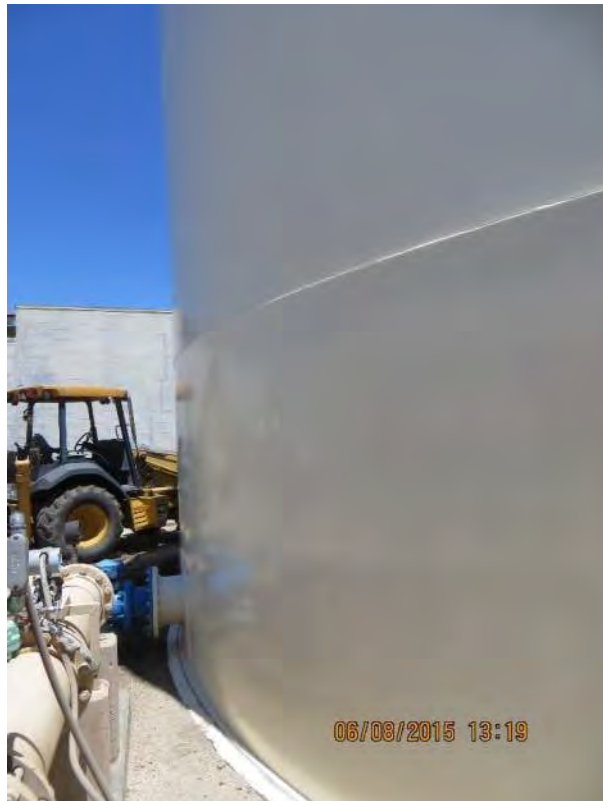
Photo 2-79: El Pueblo Tank – Area of Potential Ponding (Ground Flush with Ring Wall Footing)
