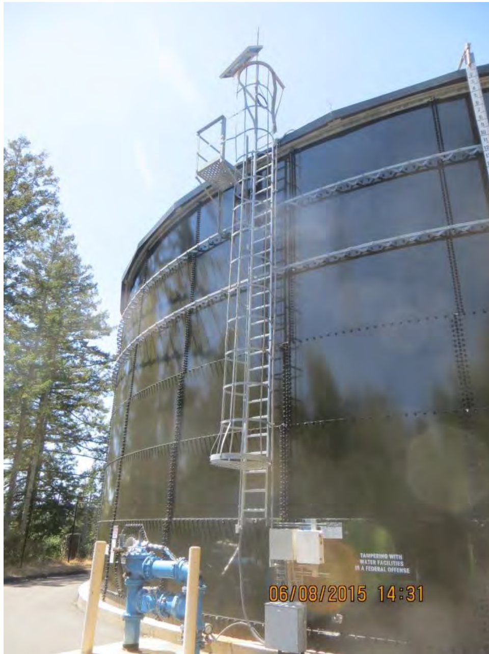
Photo 2-80: Glenwood Tank – Altitude Valve, Ladder and Telemetry System
