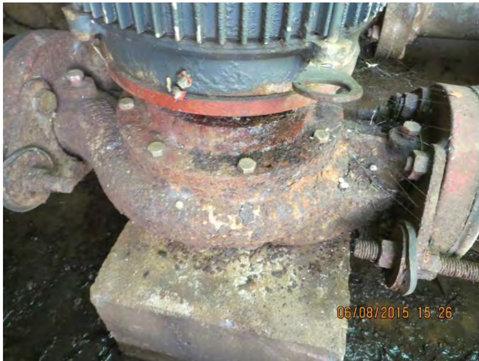
Photo 2-50: Southwood Pump Station – Corrosion on Pump Volute & Standing Water
